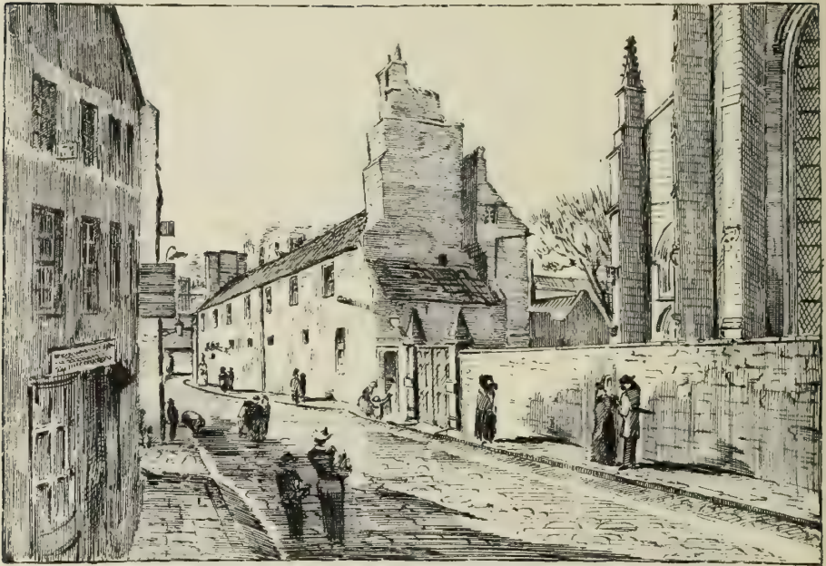
FIG. 1031.—Trinity College Church. Hospital and Part of Apse, from North-East. (From a Drawing by William Douglas, 1845.)
